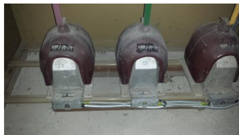
Figure 2. Photo of volatge measuring transformers during operation – no possibility to read their nameplates
